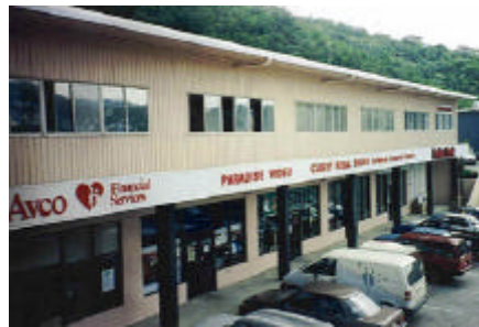
Automobile oriented buildings with little architectural detailing and extensive flat roofs are prohibited.
